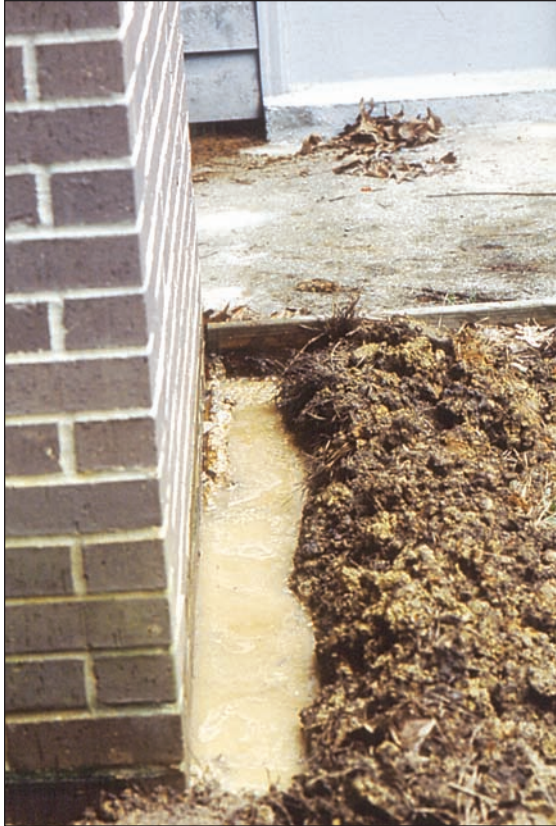
Figure 20. — Application of a chemical to soil around a foundation.
